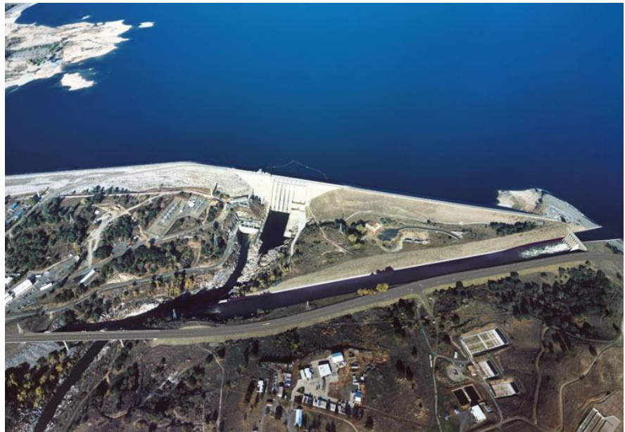
Fig. 4 new spillway is being constructed
